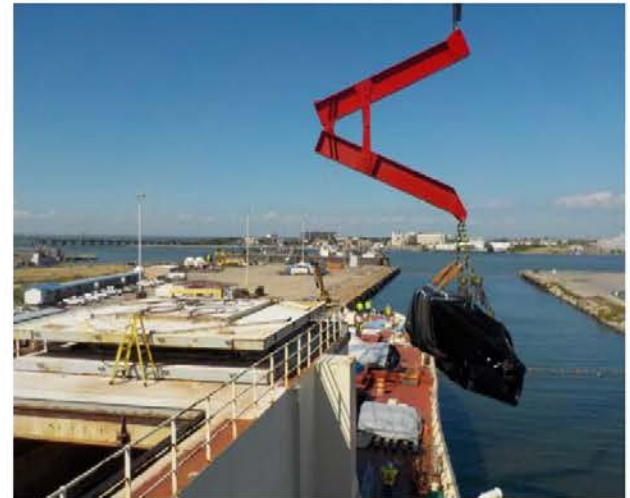
As sections of the canopy were cut into manageable pieces, the team worked to perform radiological surveys. They then packaged the pieces before they were removed and stored on the deck, pending future recycling (none of the pieces had radiological contamination and the lead can be recycled).
