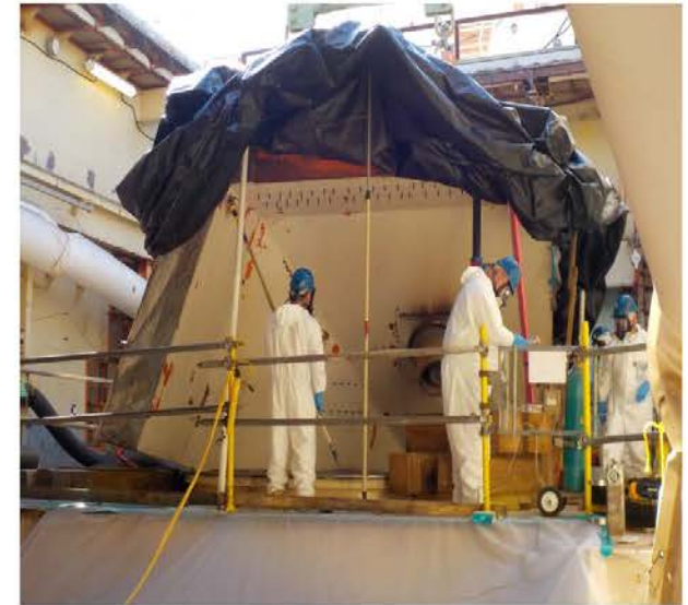
As sections of the canopy were cut into manageable pieces, the team worked to perform radiological surveys. They then packaged the pieces before they were removed and stored on the deck, pending future recycling (none of the pieces had radiological contamination and the lead can be recycled).
