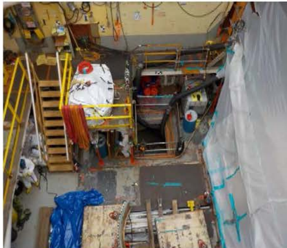
Containment (plastic sheeting and ventilation) was set up inside the Reactor Area Containment to ensure all cutting work was done safely and no lead emissions were released outside of the work area.
