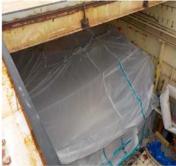
Containment (plastic sheeting and ventilation) was set up inside the Reactor Area Containment to ensure all cutting work was done safely and no lead emissions were released outside of the work area.
